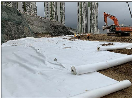
Geotextile – Formation Stability Anderson Road Development August 2017
