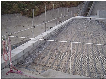
Geogrid - Reinforced Fill Wall NENT Landfill October 2005
