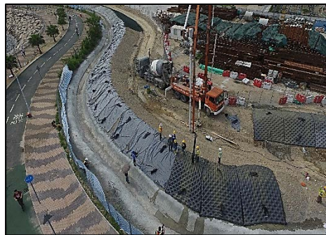
Concrete Mattress – Embankment for Coastal Protection TKO December 2017
