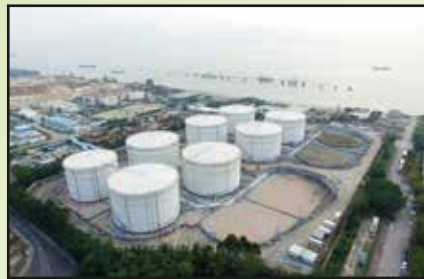
HDPE geomembrane, leak detection system, Aviation Fuel Storage Facility, May 2006 機場永久航煤儲油庫 - 聚乙烯土工膜測漏系統
