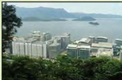
High strength woven geotextile, sand sand blanket separation, Pak Shek Kok reclamation, Dec 1998 白石角填海分隔海床和砂墊層土工布
