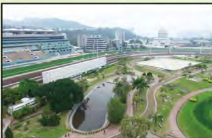
HDPE waterproofing geomembrane after 26 years, Penfold Garden, Sept 1993 彭福公園土工膜26年來防水性能良好
