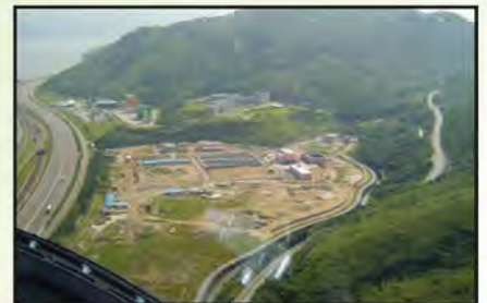
Concrete protection lining system at Siu Ho Wan treatment Works, Lantau, Dec 2004 小豪灣污水廠混凝土塚護襯裡
