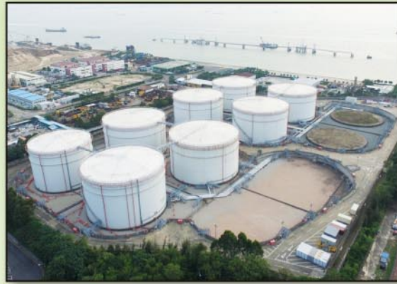
HDPE geomembrane, leak detection system, Aviation Fuel Storage Facility, May 2006
