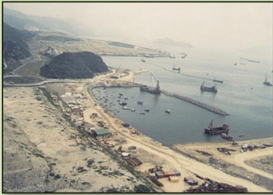
Woven geotextile, sand layer separation along seabed, TKO Reclamation, Jan 1993
