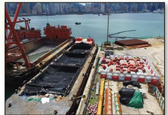
Geotextile container for contamination disposal, SCL cross harbor tunnel, Jan 2015
