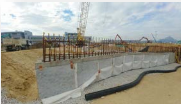
Fill slope drainage layer at HKZMB Hong Kong Link Road, July 2017 (HY/2011/09)
