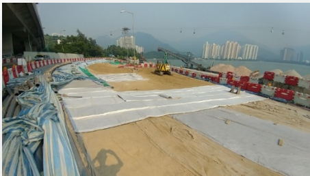
Fill slope drainage layer at HKZMB Hong Kong Link Road, July 2017 (HY/2011/09)
