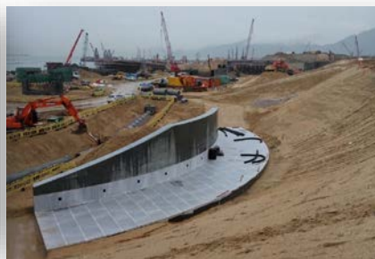
Retaining wall drainage at HKZMB Border Control Facility, March 2017 (HY/2013/03)
