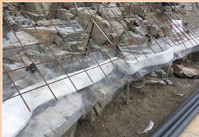
Relief drain at Anderson Road Quarry Development
