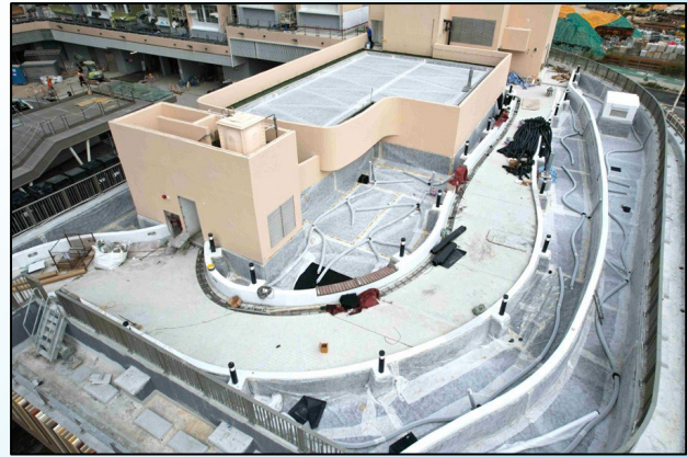
Filter Fabric, PHD at Anderson Road Quarry Site, March 2024 (HKHA20190293)
