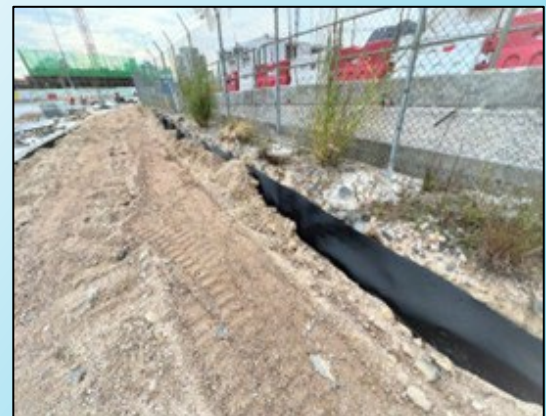
Root Barrier, Anderson Road Quarry, October 2022 (NE/2016/01)
