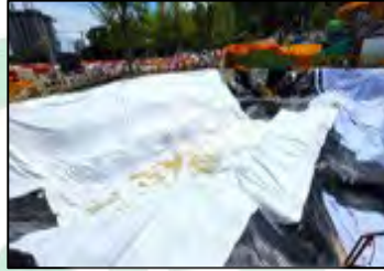
HDPE membrane protection (NL/2020/06)
