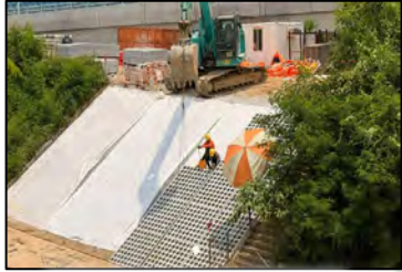
Ground cover to Grasscrete (ND/2019/04)
