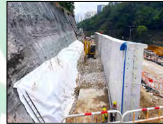
Rockfill filter layer (NE/2017/03)
