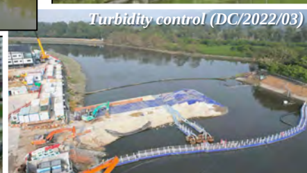
Encasing seawall work (WENTX Landfill)
