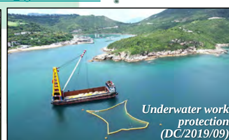
Marine piling silt curtain (C24W08)
