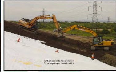
Enhanced interface friction for steep slope construction
