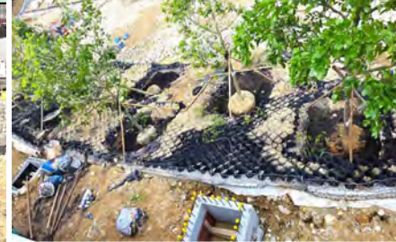
Soiling and planting work
