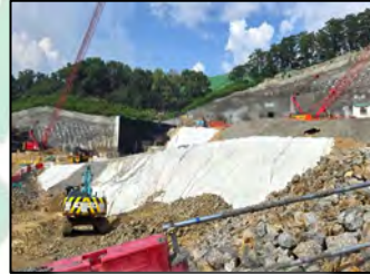
Rockfill separation (WENTX Landfill)
