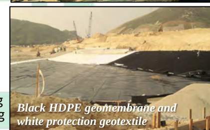
Geomembrane lining system
