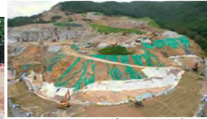
Separation formation and backfilling (CV/2022/11)
