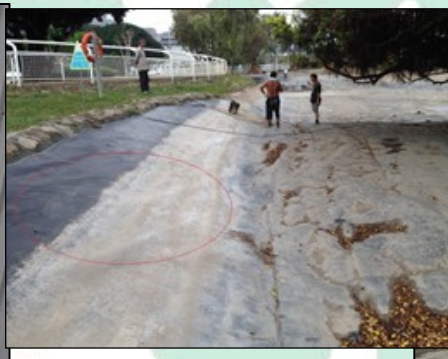
Penfold Garden desilting and cleaning
