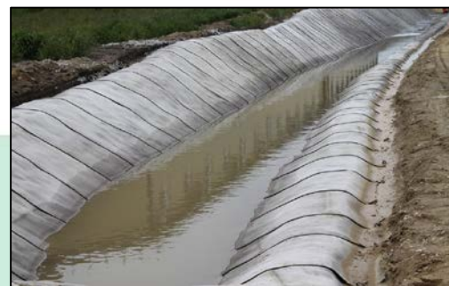
Channel lining surface application
