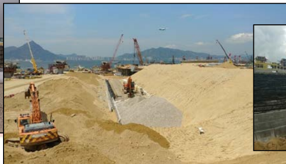
Backfilling in operation
