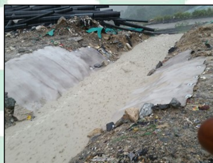
Channel lining trial at WENT Landfill
