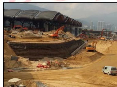
Facing with planting medium sand bag to support vegetation
