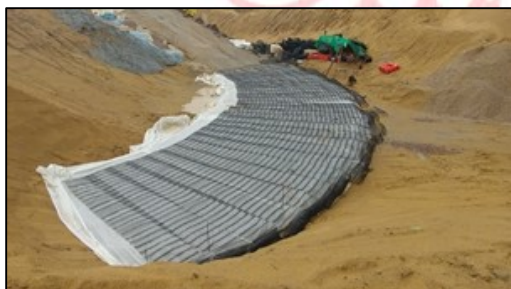
Geogrid changes direction in construction
