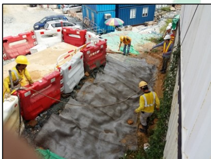
Erosion protection trial at Liantang
