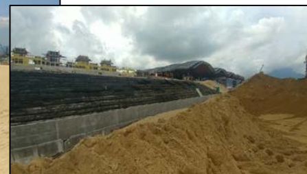
Facing with planting medium sand bag to support vegetation
