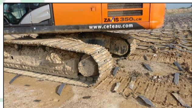
PVD run over by excavator
