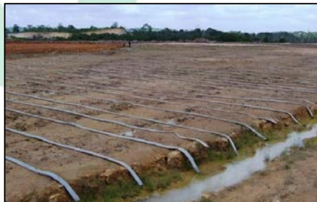
Strip drain to drainage system
