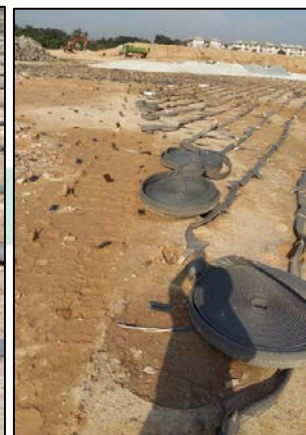
Installation of PVD
