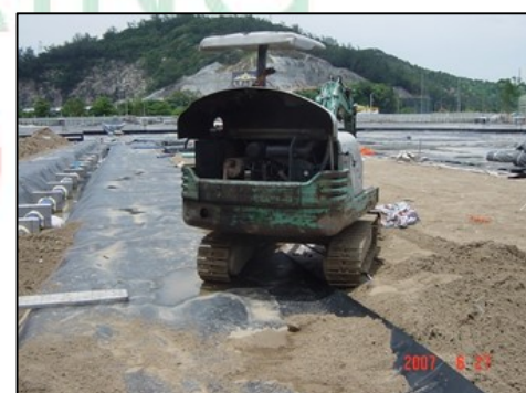
PVD run over by excavator
