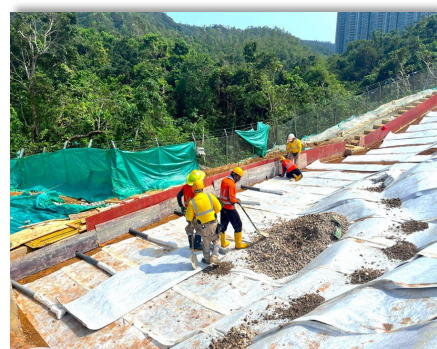
Fill Slope Drainage at TKO – Yau Yue Wan, October 2023 (CV/2021/04)
