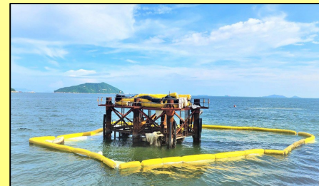
San Shek Wan Sewage Treatment Works, August 2023 (DC/2020/02)
