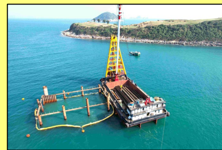
Provision of village Sewerage Sai Kung, January 2024 (DC/2019/09)
