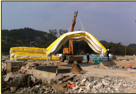
Handling of the silt curtain
