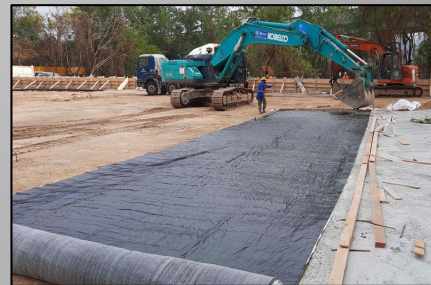
Wetland Waterproofing, Development of Lok Ma Chau Loop, January 2022 (YL/2020/02)
