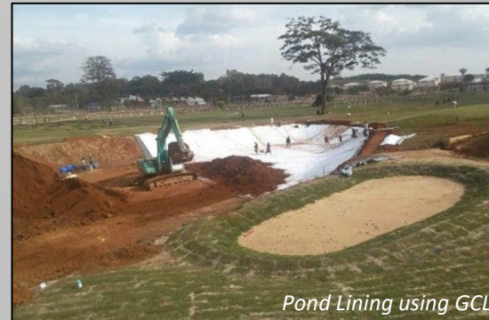
Installation of GCL
