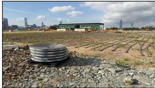
Ground consolidation treatment Lok Ma Chau Loop, June 2019 (YL/2017/03)
