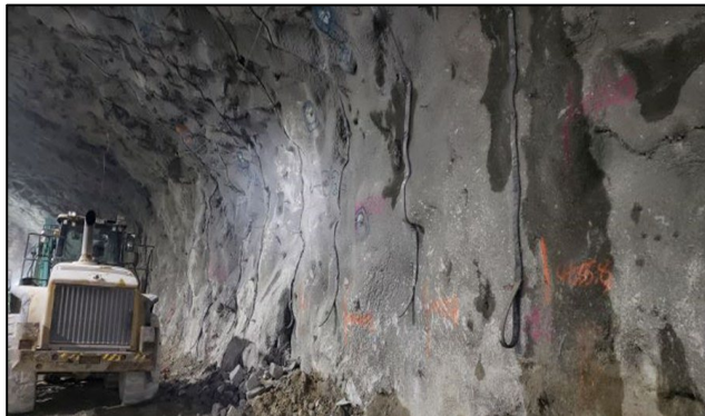
Tunnel Drainage, Shatin Sewage Treatment Works to Caverns, November 2020 (DC/2018/05)
