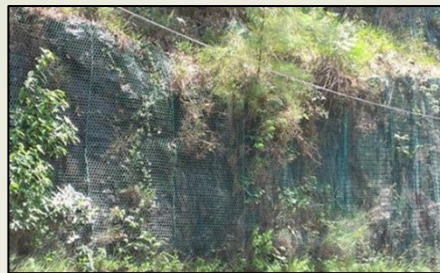
Erosion Control at Tolo Highway August 2012
