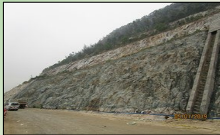
Erosion Control at Anderson Road Quarry, March 2019
