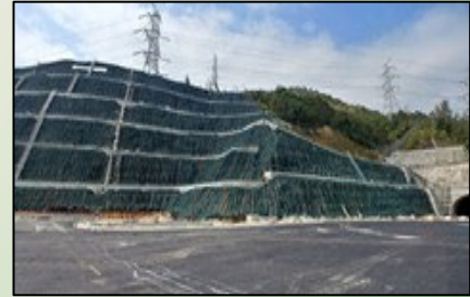
Erosion Control at Tuen Mun Chek Lap Kok Link, March 2018
