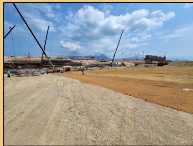
Third Runway Concourse May 2022 (C3405)
