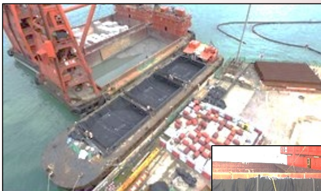
Disposal of type 3 marine sediment at Shatin to Central Link – NSL Cross Harbour Tunnel, October 2016, SCL1121
