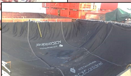
Disposal of type 3 marine sediment at Shatin to Central Link – NSL Cross Harbour Tunnel, October 2016, SCL1121
