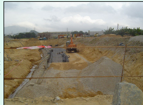
Vertical river embankment along Shenzhen River, 2003
