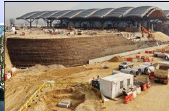
Embankment at HKZMB BCF Vehicle Clearance Plaza, HY/2013/03, 2017
