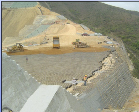
Embankment at NENT Landfill, 2005
