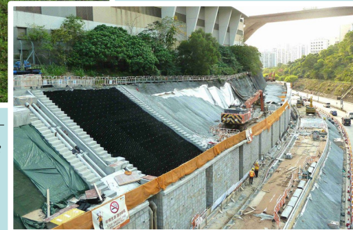
Soil Retainment for Landscaping on slope – Anderson Road Quarry Site – Road Improvement Works. March 2025 (NE/2017/03)
