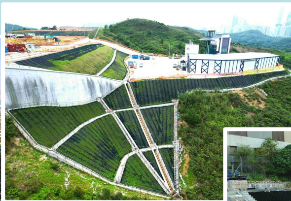
Soil Retainment for Landscaping – Site Formation and Infrastructure Works at Kong Nga Po. March 2023 (ND/2018/01)
