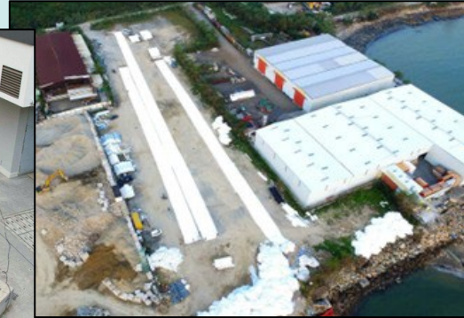
Sand Blanket Separation (C3205)
