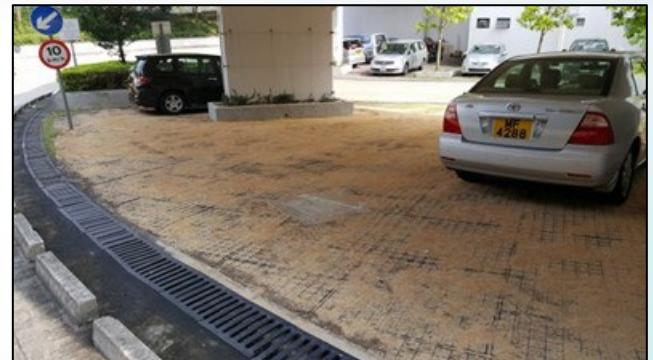
Landscape Paving for Fire Access at Shatin Transfer Station, May 2017 (EP/SP/76/14)
