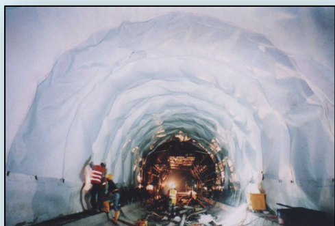
Lam Tin Tunnel February 2001
