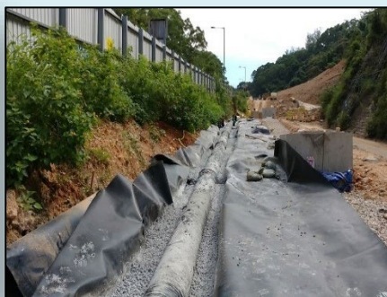
Hiram's Highway November 2018
