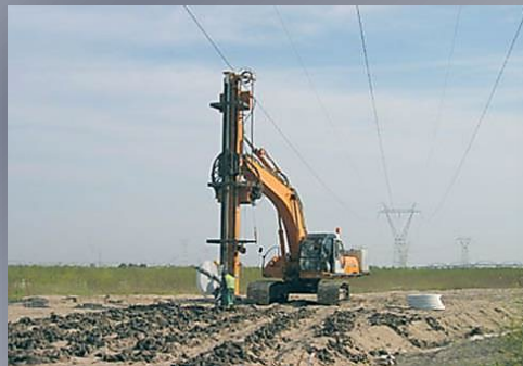
Telescopic rig operation under flyover, 14m installation with head clearance of 8m.
