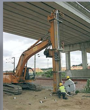
Telescopic rig operation under power lines, 18 m installation with 12 m head clearance.
