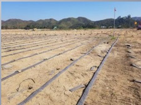
Ground consolidation treatment
