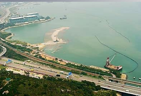
Hong Kong-Zhuhai-Macau bridge – Hong Kong Link Road – Scenic Hill. Jan 2013 (HY/2011/03)
