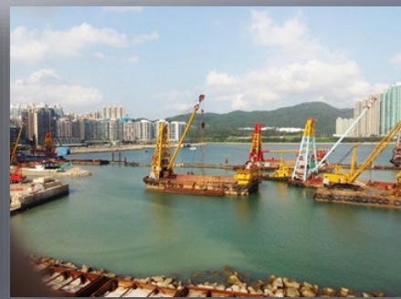
Tseung Kwan O - Lam Tin Tunnel Road P2 and Associated Works, April 2019 (NE/2015/02)
