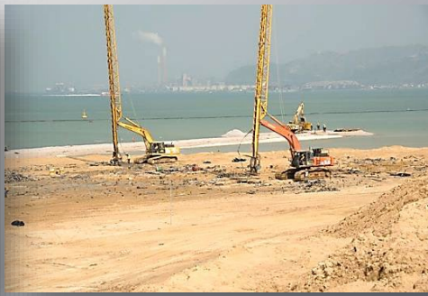
Hong Kong-Zhuhai-Macau bridge – HK Boundary Crossing Facilities. Feb 2014 (HY/2010/02)
