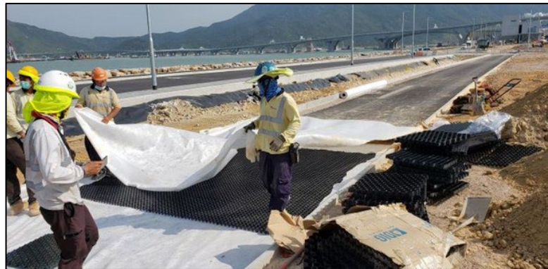
Drainage layer at Tuen Mun – Chek Lap Kok Link August 2020 (HY/2017/10)
